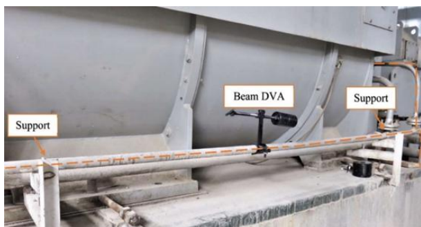
Figure 4. Beam DVA installed on Lube oil piping
