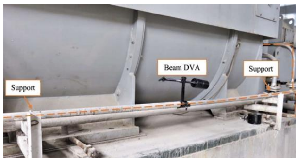
Figure 4. Beam DVA installed on Lube oil piping
