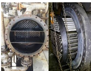
Figure 1. Replacement of the heat exchanger tube bundle at the Shiraz refinery
